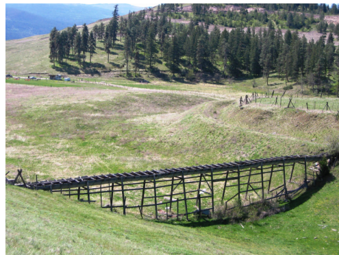
BMID Trestle Flume (1948-1970)
