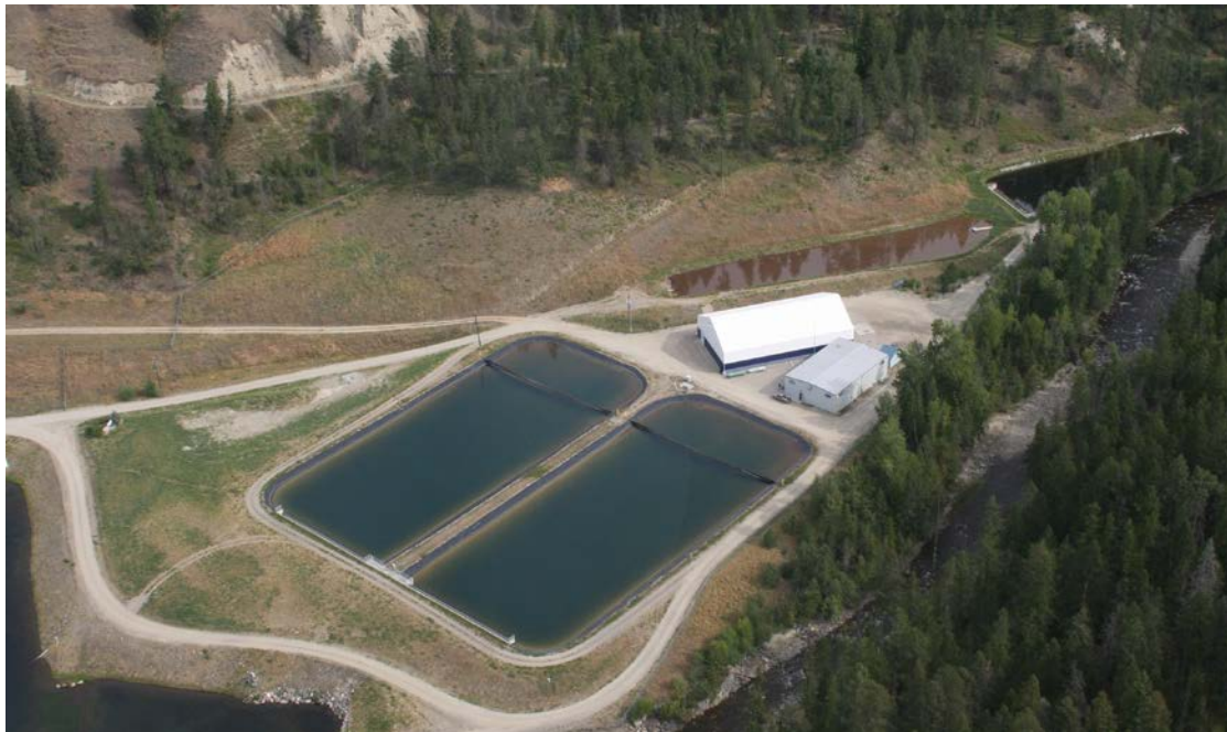
Figure 1.1 BMID Water Treatment Plant (note new Guard-All Building)
