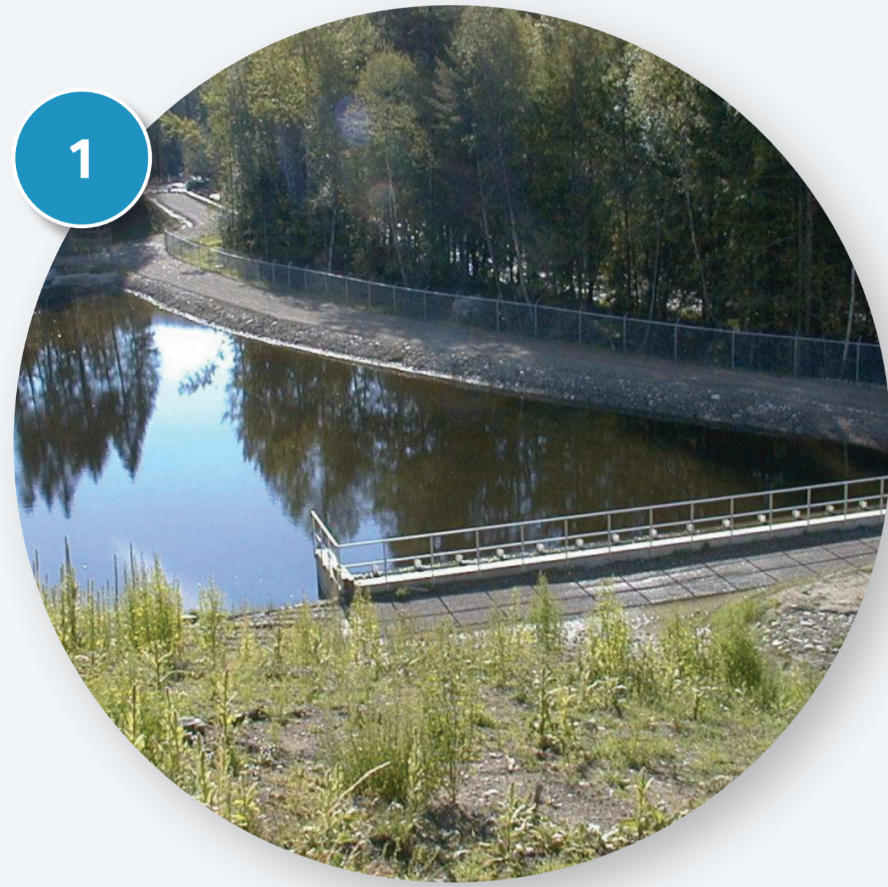
1 Automated Headgates and Grit Pond
