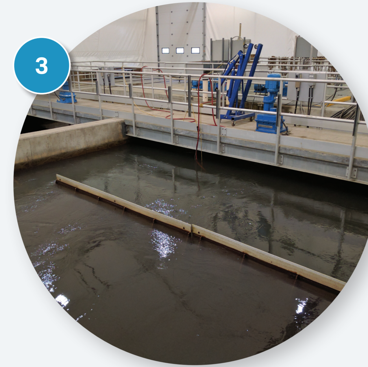
3 Rapid Mix and Floc Tanks
