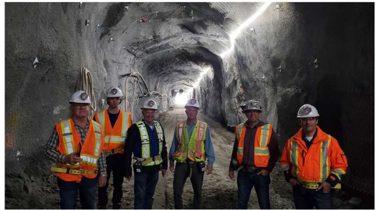
Photo - Trans-Mountain Pipeline Tunnel -2024 (same end section size as BMID Tunnel Extension)
